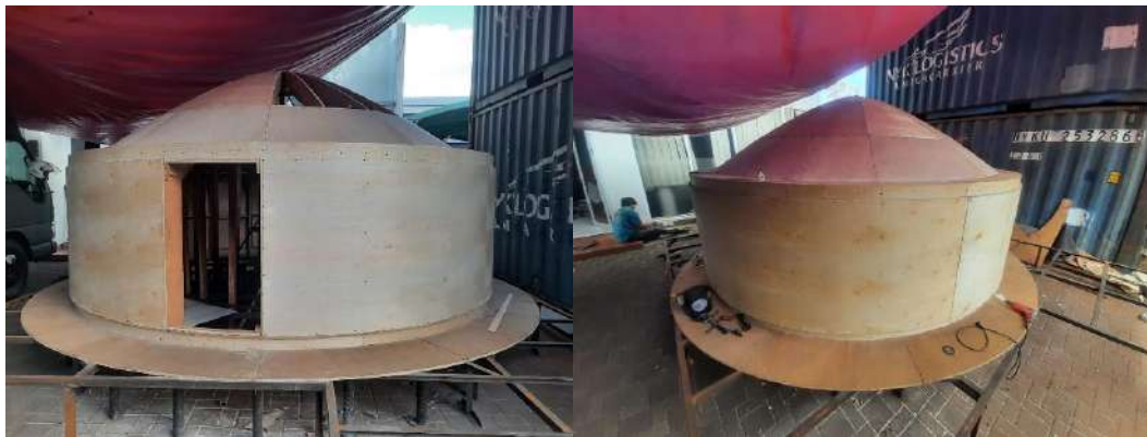
Gambar 6.6 Proses penutupan rangka moulding FECABS
