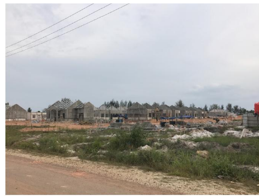
Figure 11 Construction of Military Housing in Natuna
